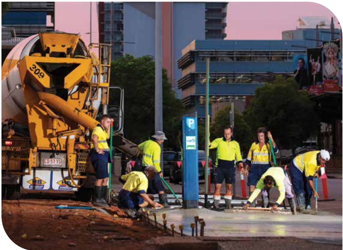
CITY OF DARWIN STREETScape BEAUTIFICATION PROJECT 2020
